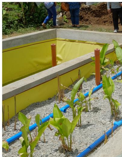
Vertical subsurface flow constructed wetlands.
