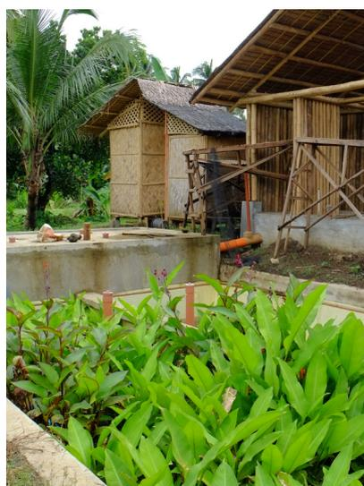
Horizontal subsurface flow constructed wetland.
