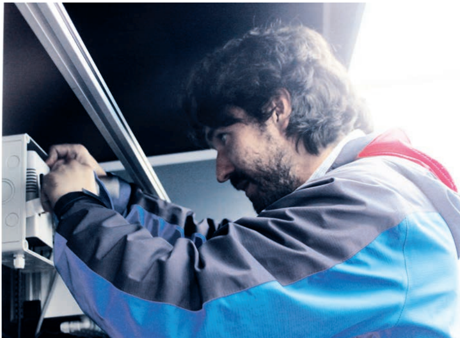
Fudación Humedales Team Trained to Maintain Filtering Unit
