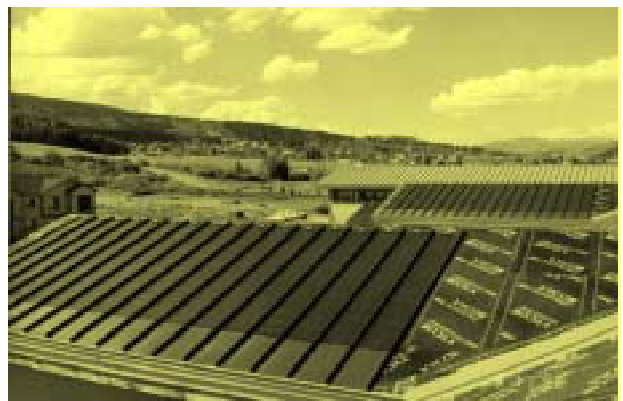
Solar cells have been directly installed as part of this building's roof (courtesy NREL).
