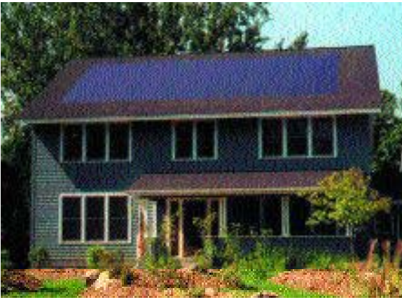
A solar-powered house
