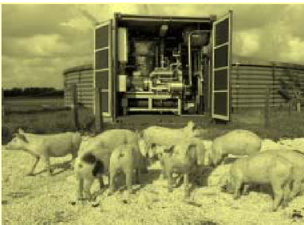
A biogas plant converts animal manure into biogas
