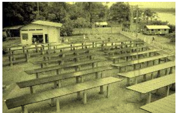
PV modules can often be wired together to generate larger amounts of solar power.
